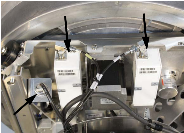
Figure 8-97: Disconnecting the LNBS
