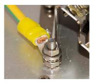
Figure 6: Grounding Bolt
