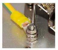
Figure 8: Grounding Bolt
