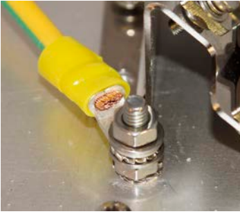
Figure 8: Grounding Bolt
