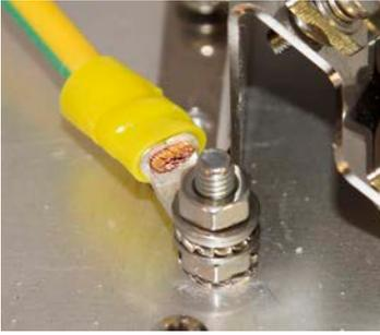
**Figure 8: Grounding Bolt**
